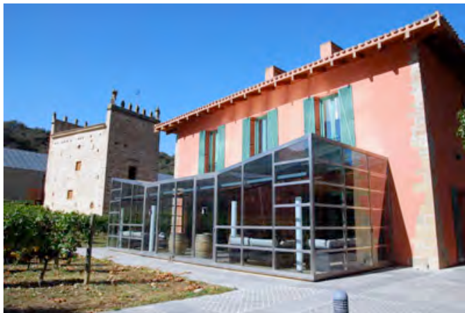
Tower and tasting room.
